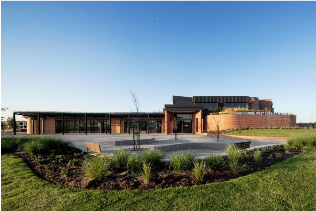
Figure 1: Cranbourne West Community Hub
