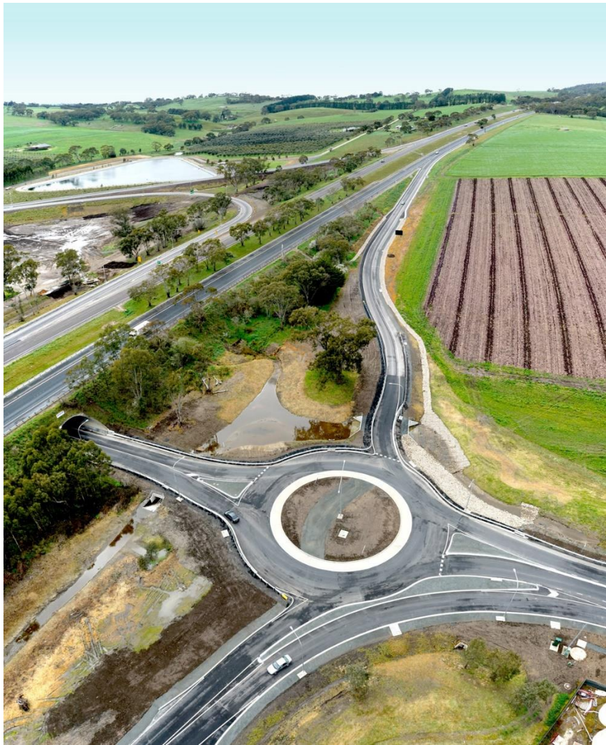
Figure 18: Aerial view of the Bald Hills Road freeway interchange
