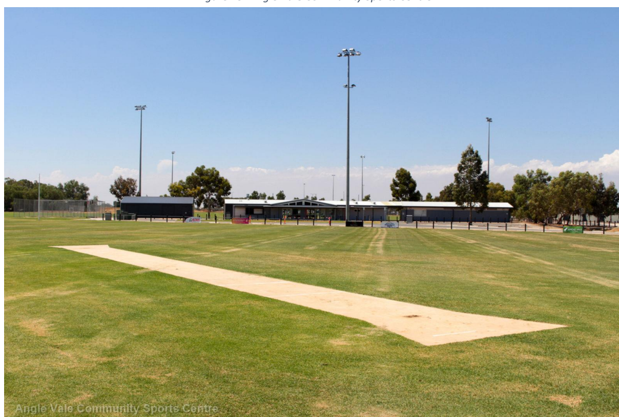
Figure 23: Angle Vale Community Sports Centre
